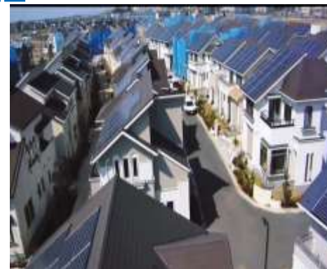
sostres solars i NZEB
