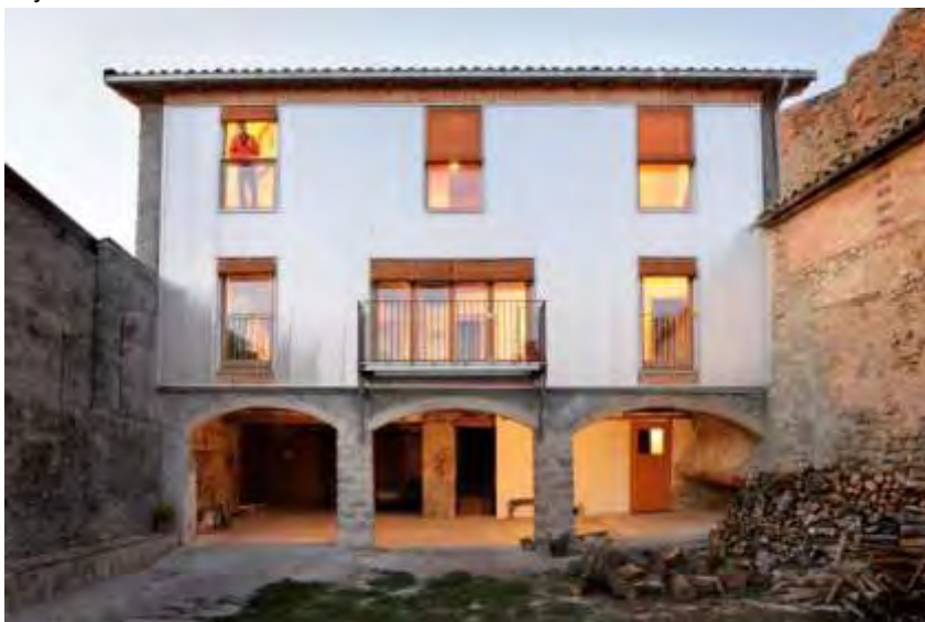
South façade of polycarbonate panels of 8 layers
